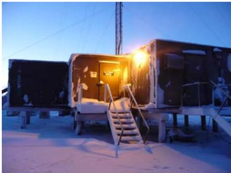
**FIGURE 4.** Proper Shelter Installation on Permafrost
